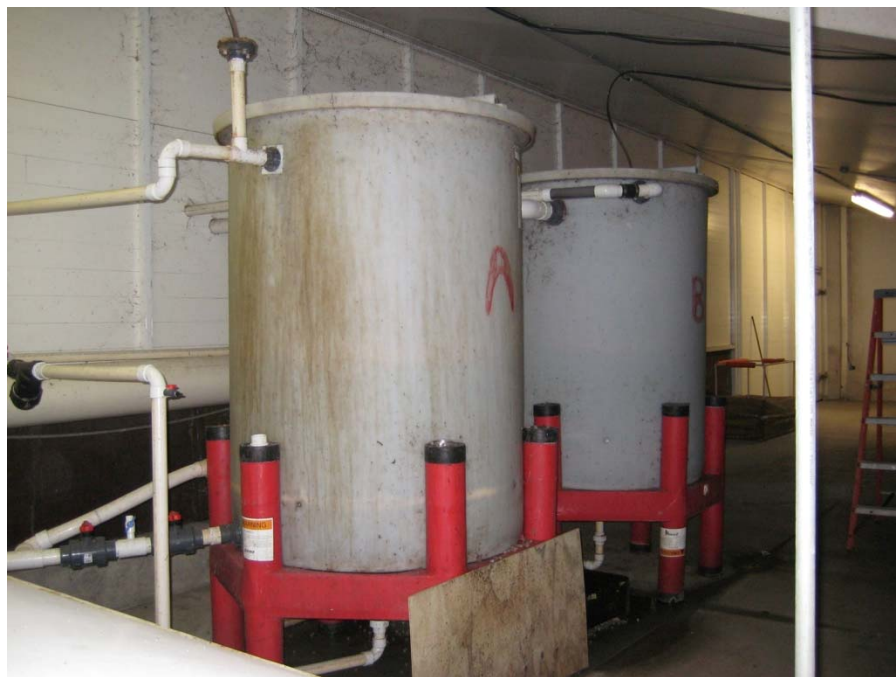
Figure 9 Anaerobic Denitrification Reactor
